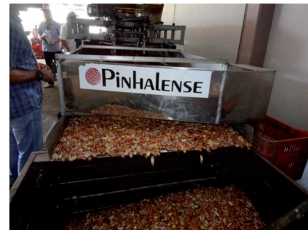
Illustrative photos of the equipment installed
